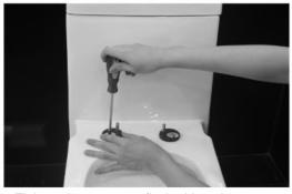
2. Tighten the screws to fix the hinge bases (but not fully tightened at this stage)
