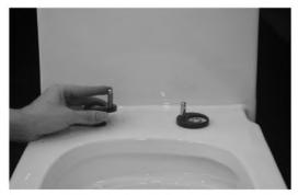
Insert the screws on the hinge base and then into the holes on the pan.
